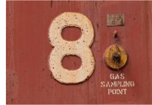
Gas sampling point.
